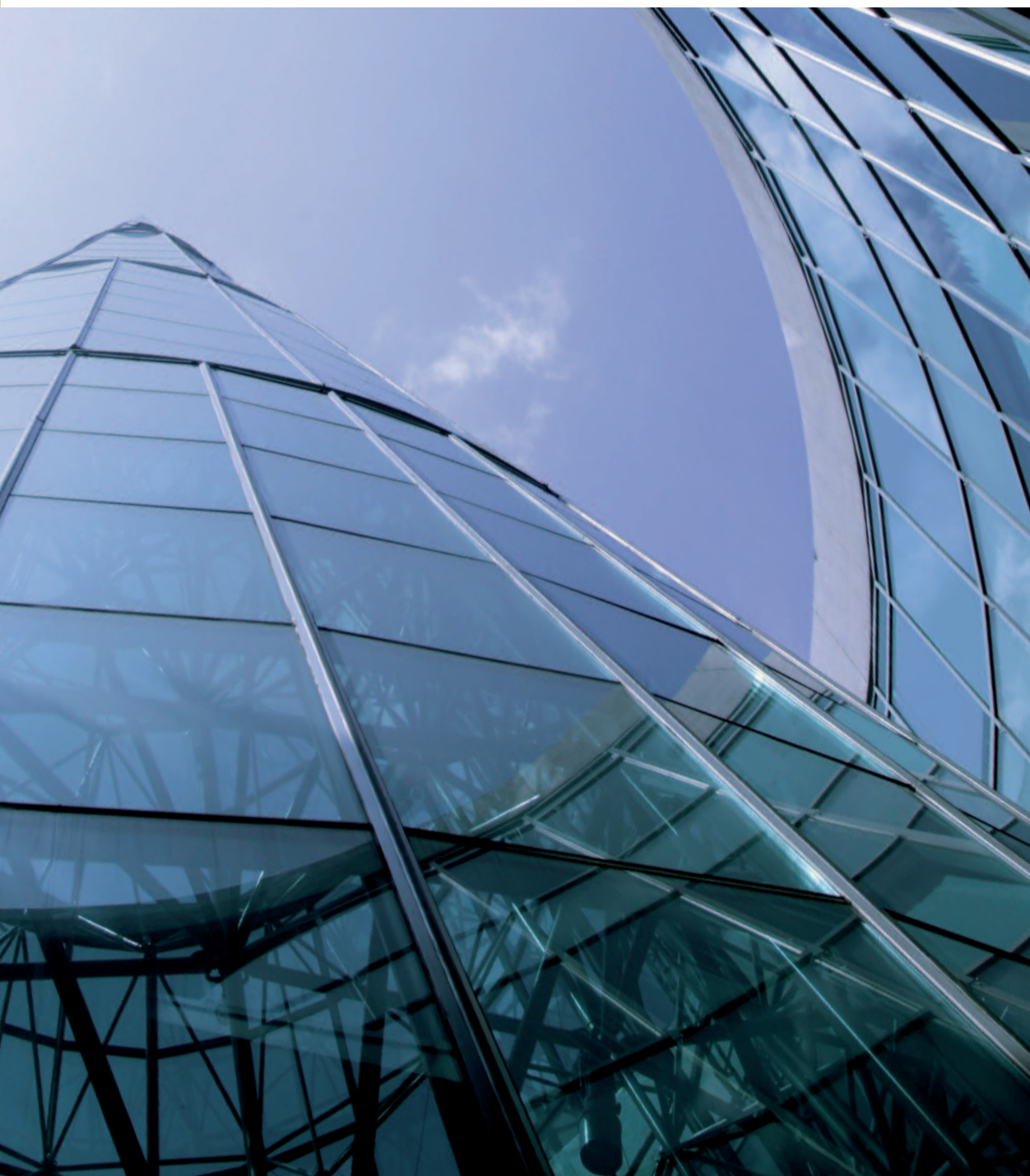
Wheelock Place Exterior
